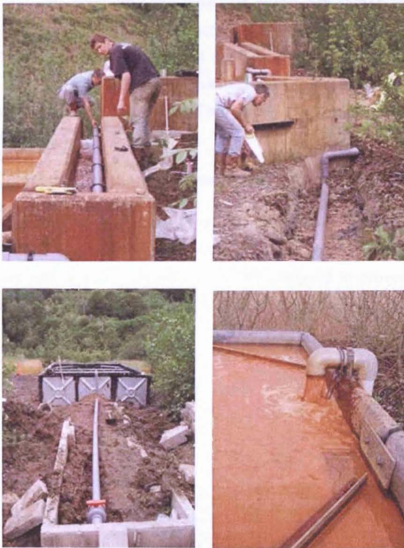
Figure 4-24: Sequence of photographs showing the feed pipe from the distribution weir to the VFR inlet
