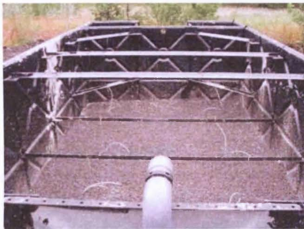
Figure 4-18: View facing west of the finished plenum floor with the 100 mm thick bed of 20 mm sandstone gravel.
