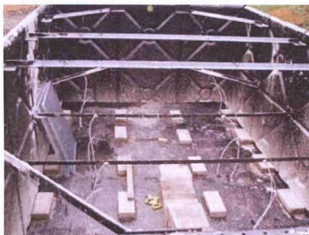
Figure 4-17: View facing west of the concrete block support arrangement for the plenum floor
