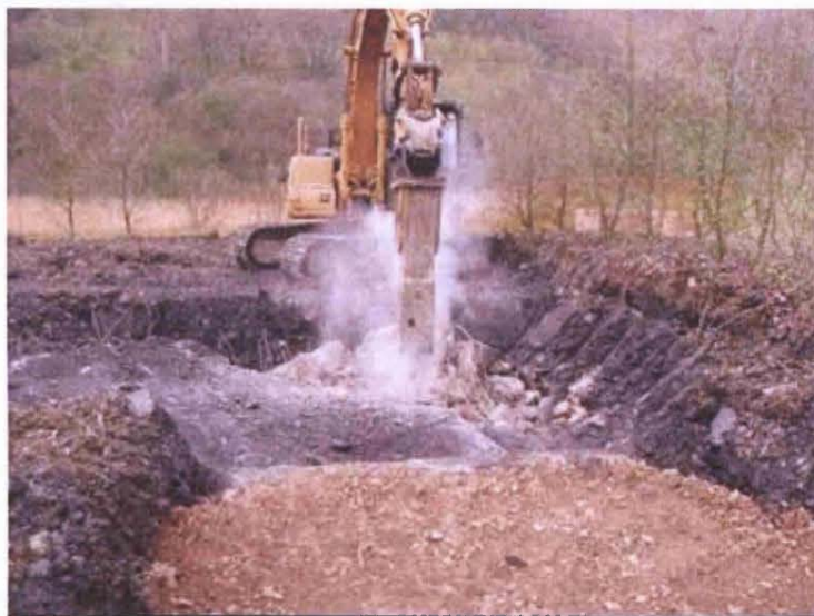
Figure 4-10: View looking west across the excavation showing the use of the pneumatic hammer to break the reinforced concrete slab.
