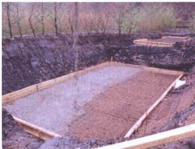
Figure 4-13: View facing east during the first pour of concrete onto the sub-base, shuttering-mesh assembly.
