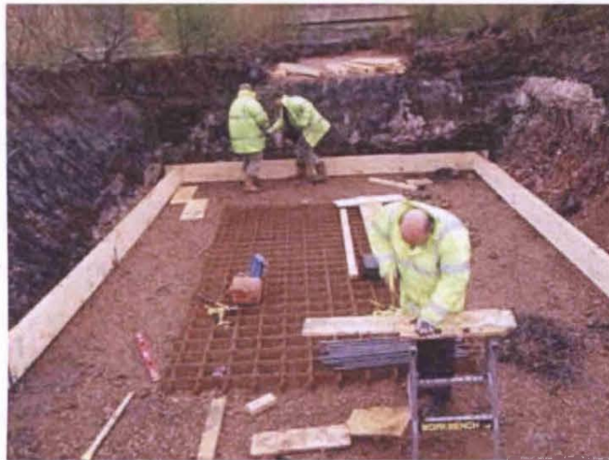
Figure 4-12: View facing east of the assembly of the ply-wood shuttering, ready for layering of the reinforced mesh and concrete pour.
