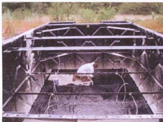
Figure 4-16: View facing west of the inside of the tank after the second concrete pour The concrete is being coated with bituminous paint to minimise seepage. The sample tubes can clearly be seen protruding from the concrete base. Photograph courtesy of Dr Devin Sapsford.
