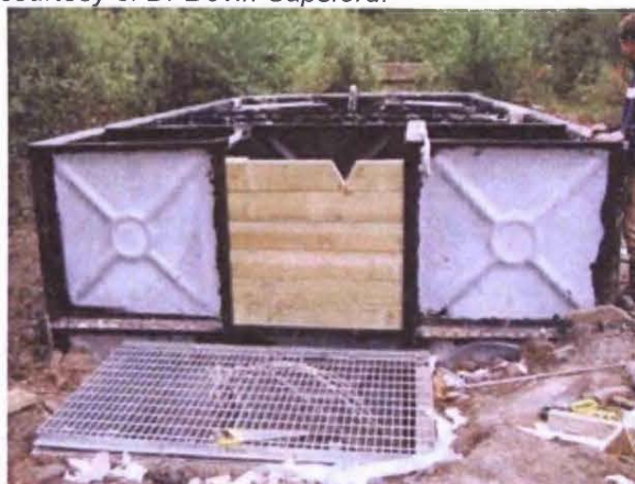
Figure 4-22: View looking east of the finished discharge chamber showing the galvanised steel grating.
