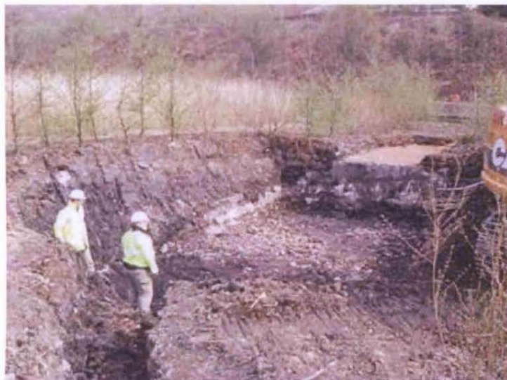
Figure 4-11: Looking east across the finished excavation ready for delivery of Type 1 sub-base.
